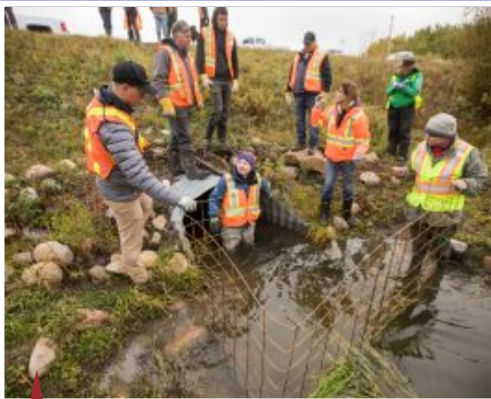
Volunteers work to install a barrier to prevent beavers from damming the water flow around a culvert near Priddis on Sept. 23.
