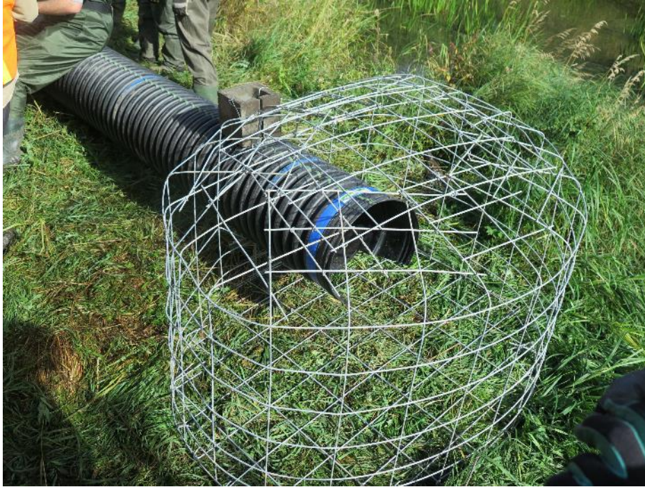
Figure 5: View of the intake end of the pond leveller after being constructed on land, prior to installation in the pond.
