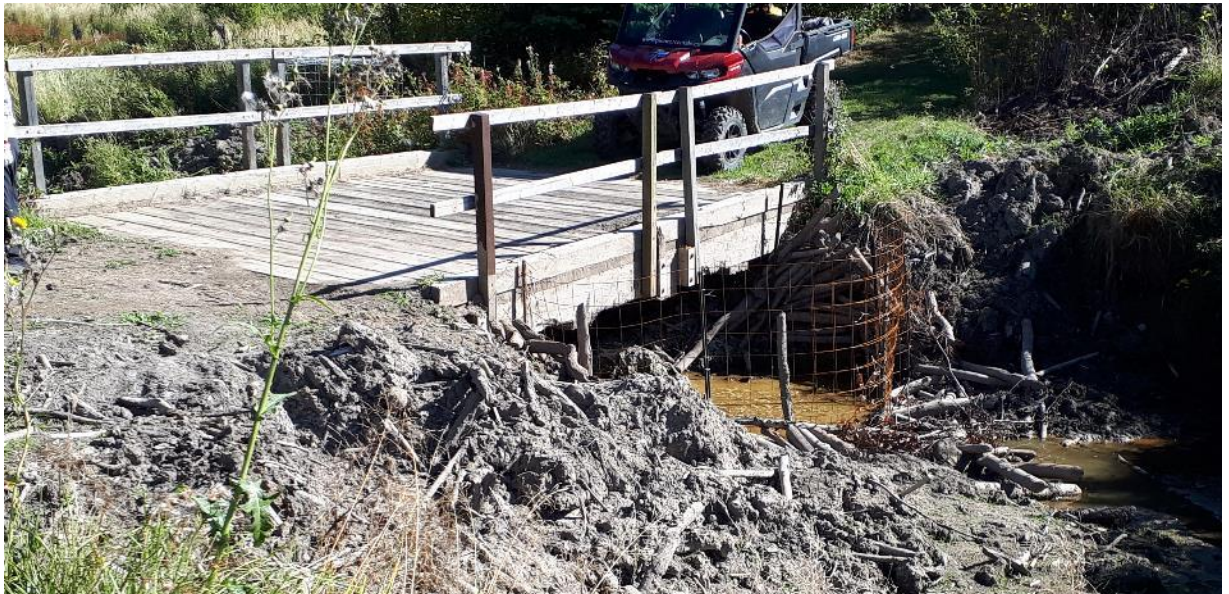
Figure 15: Modification of the diversion dam fence concept used on a bridge (Location: Cooking Lake Blackfoot Provincial Recreation Area, Alberta)
