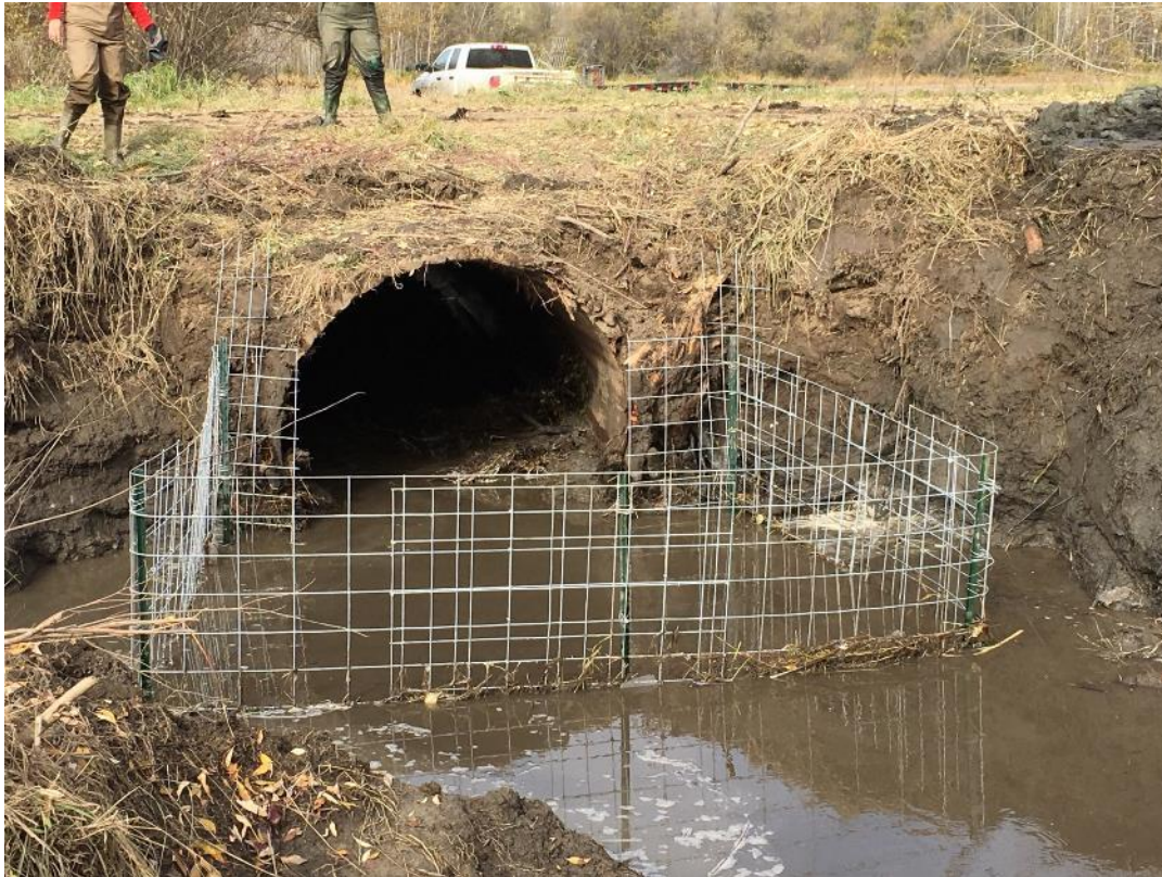
Figure 9: Culvert protector installed on a 6' culvert (Location: County of Barrhead, Alberta).
