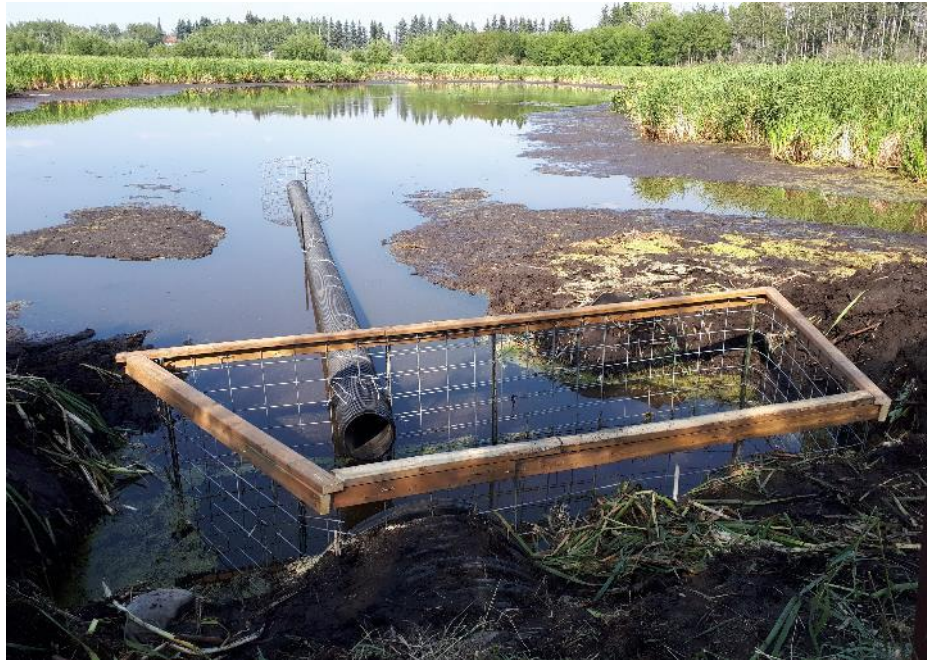
Figure 12: A second example of a combination device (pond leveller and culvert protector) (Location: Lamont County, Alberta).
