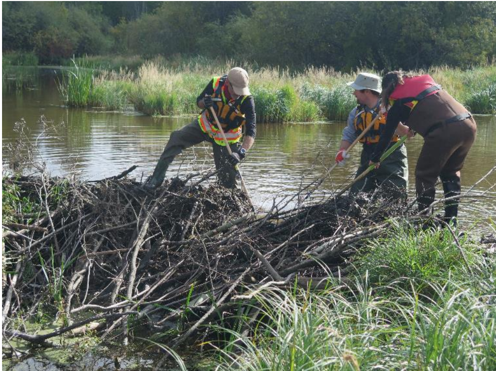
Figure 2: A second example of practitioners creating a notch in a beaver dam prior to installing a pond leveller (Location: Lac Ste. Anne County, Alberta).
